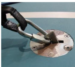
Maillon attaching floor sling to floor anchor
